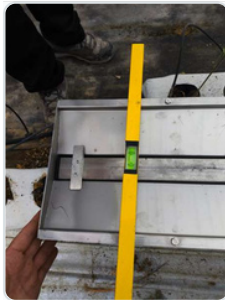
Leveling the width of the tray
