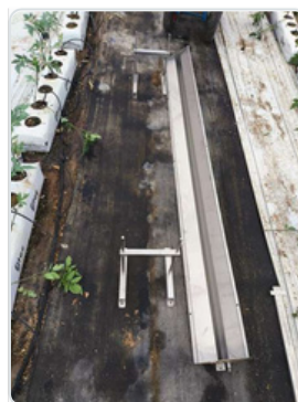
Tray affixed to the supports with screws.
